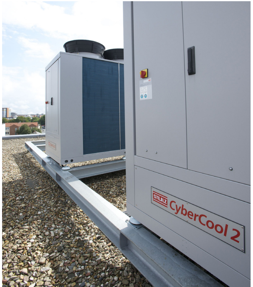
CyberCool 2 chillers with Indirect Free Cooling
