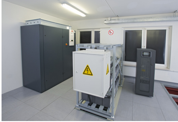
Equipment room 1 with CyberAir 3PRO CW and UPS
