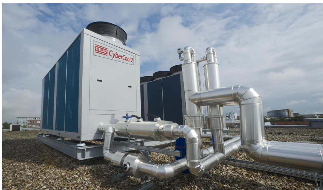
AxiTop fan diffuser attachments provide additional noise reduction.
