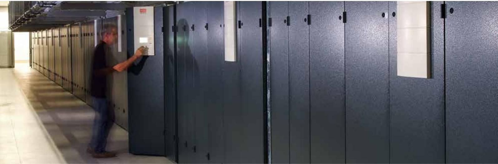
STULZ CyberAir 3 allows for both central and distributed arrangement of air conditioning units. Every unit has its own intelligence. Up to 20 units work together in the system network.
