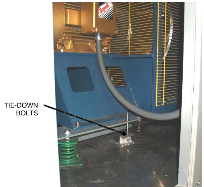
Figure 5. Blower Tie-Down Bolts
