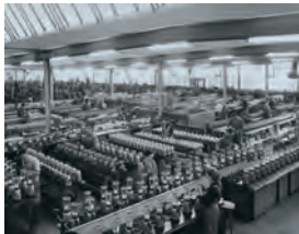
Foundation of the "ALBERT STULZ Electrical Appliance Factory"
