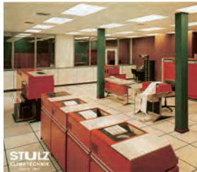
STULZ specialized in mission critical cooling.
